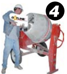
4 With mixer still turning, add pre-determined units of DOTline™. Mix for 1 minute
