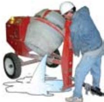
2 DO NOT drain into repair site!
