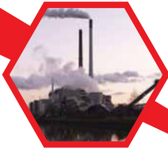
Coal Burning Utility
