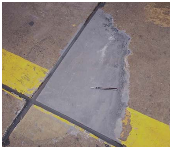
Figure 7: Repair completed using Pavemend
