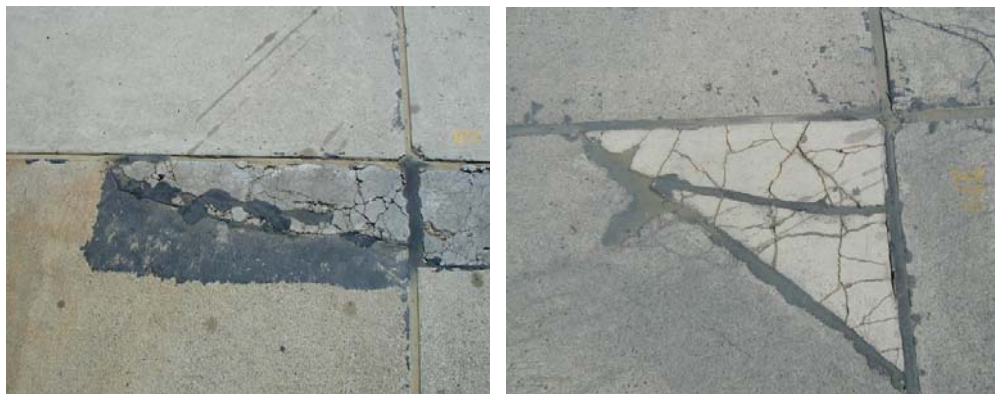
Figure 4: Deterioration process of cement based materials due to sudden ambient temperature changes
