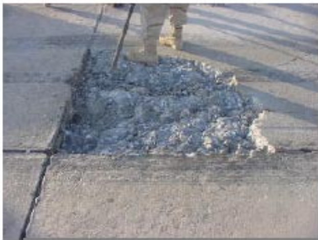
(a) Before completion of emergency repair..
