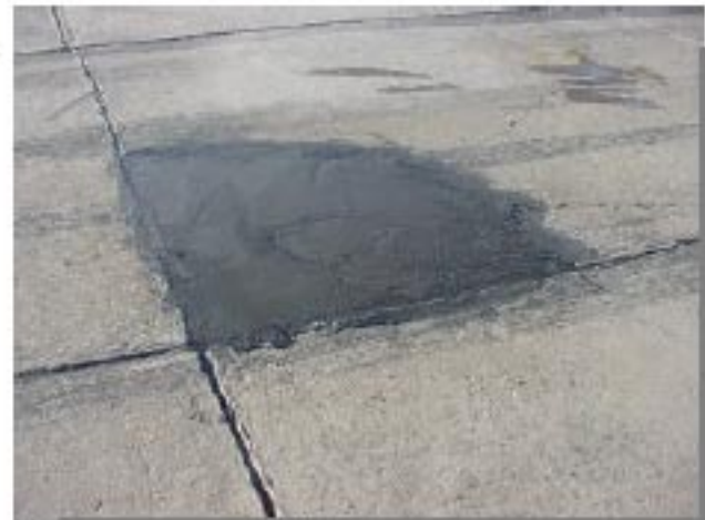
(b) After completion of emergency repair.
